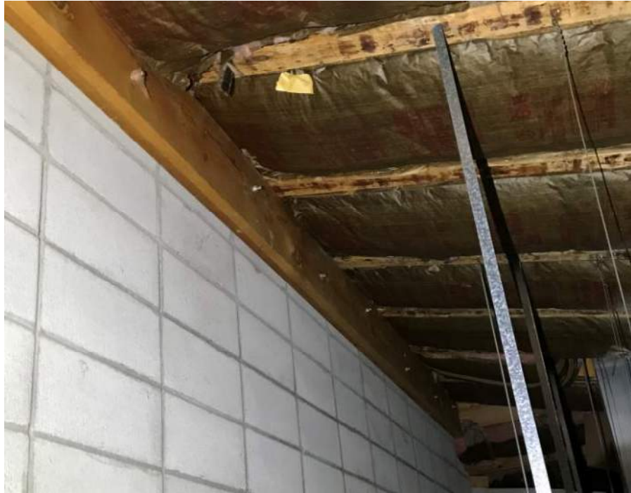
Figure 9. TJI Joist Support at Interior CMU Wall (1985 Classroom Addition)
