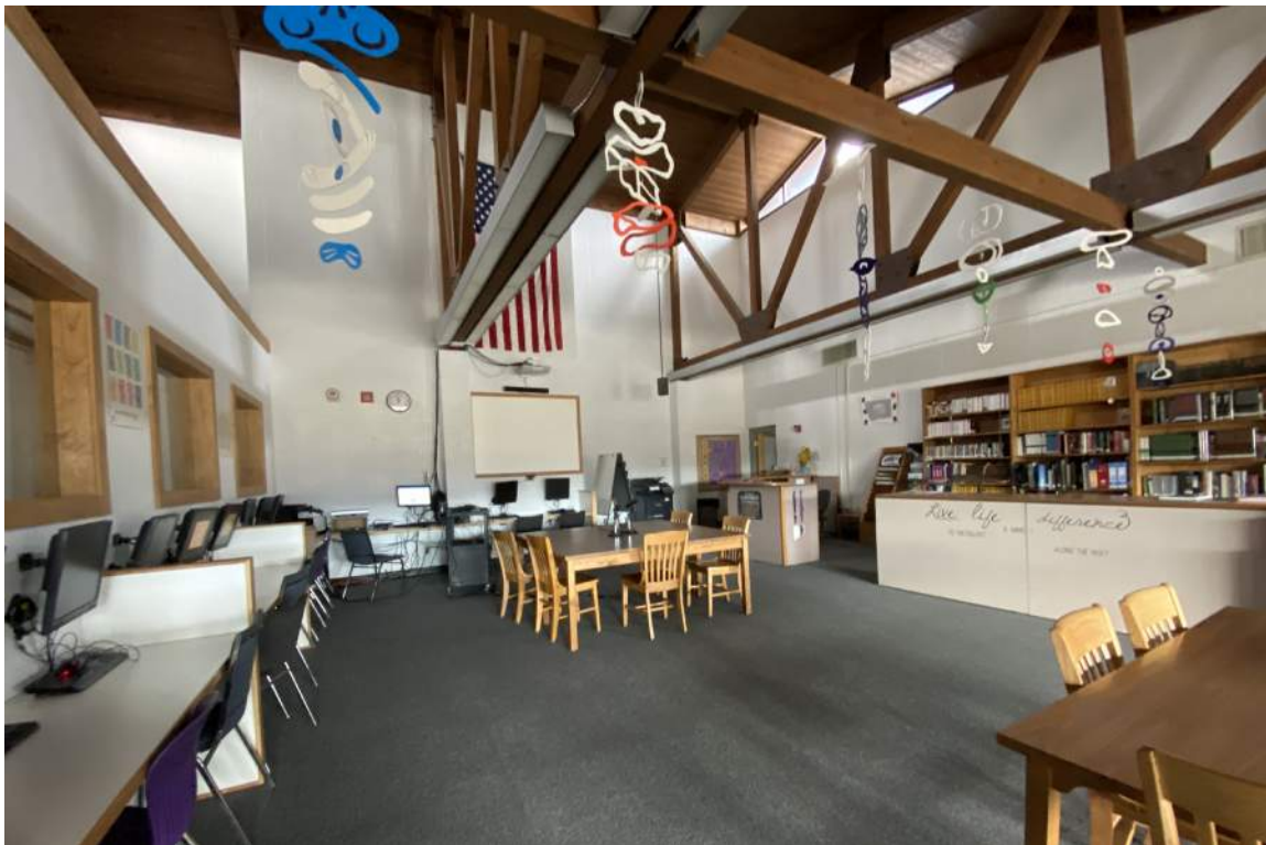
The library space with exposed wood trusses.
