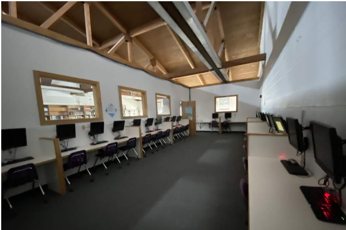
View of computer lab within library space. The large gap above the walls allows sound to travel between spaces.
