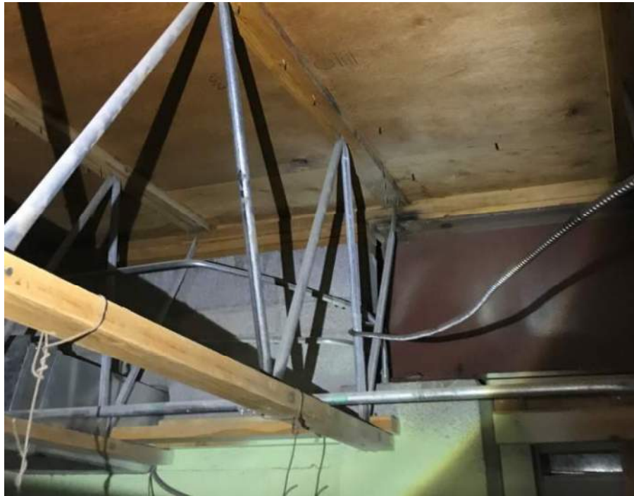
Figure 8. TJL Bearing on Interior CMU Wall (1974 Classroom Addition)
