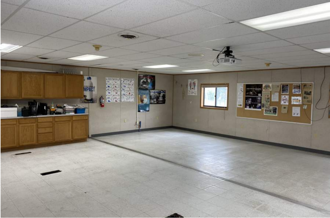
Another modular classroom. Maintenance has been kept up in these rooms and they have floors, ceilings, and casework in good condition. ■
