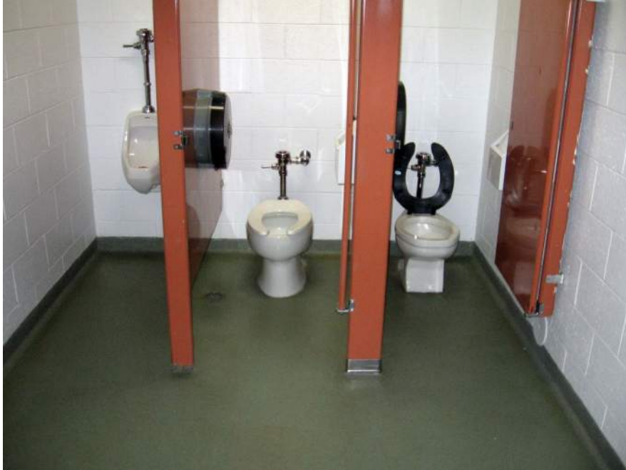
M3: Old Gym Area Rest Rooms
