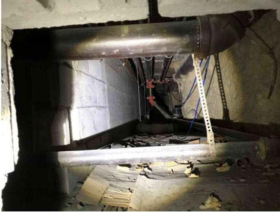
Figure 17. Maintenance Tunnel Under 1956 Gym Floor
