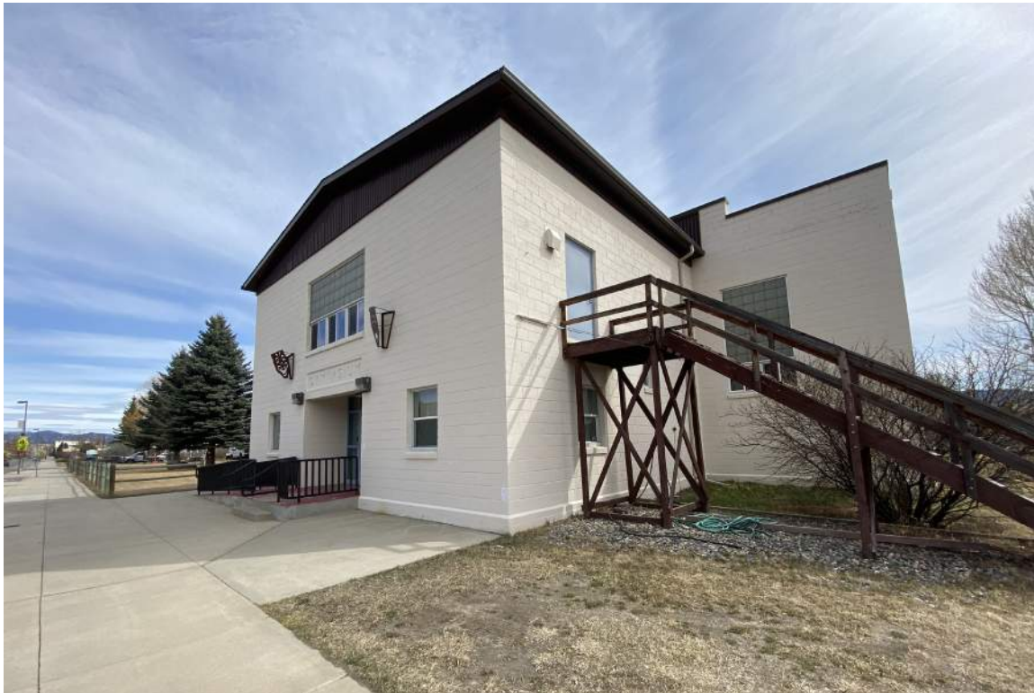
West entrance at existing gym and Art Room, facing Main Street. The entrance is very close to the street edge. Art Room egress stairs are on the right.
