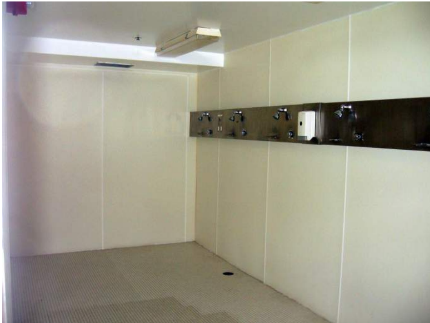
M6: Lower Level Locker Room Showers
