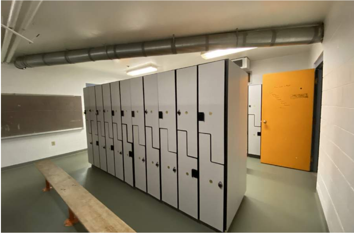
Women's lockers in the lower level of the Existing (South) Gym area. These locker rooms were reported to have issues with accessibility, ventilation, and adjacency to the Men's locker room. These are only accessible by stair.
