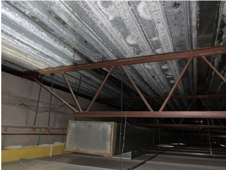
Figure 3. Roof Framing Above Wrestling Room (1985 Addition)
