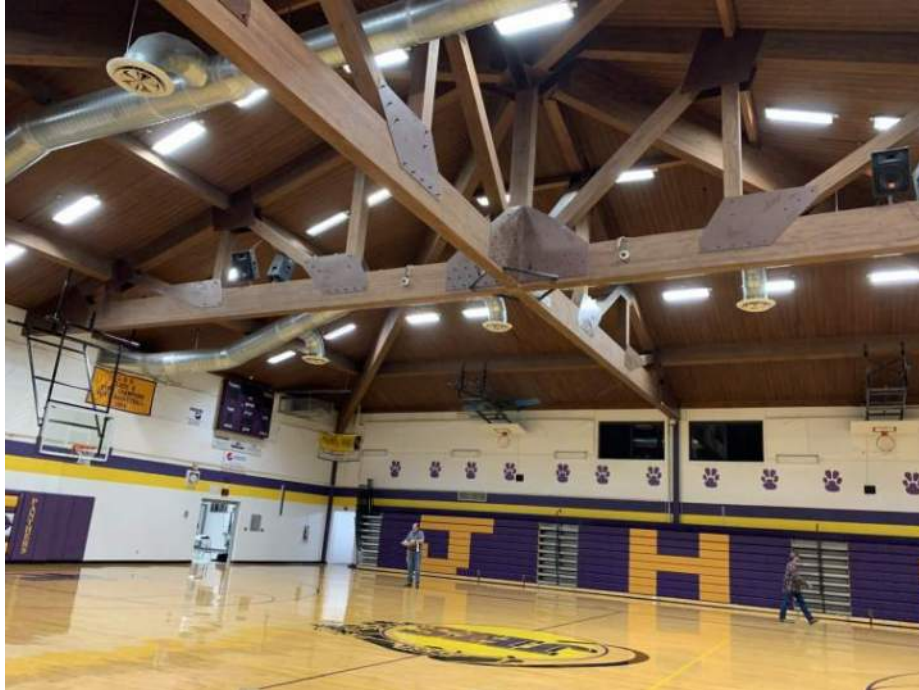
Figure 2. 1985 Gym Roof Trusses
