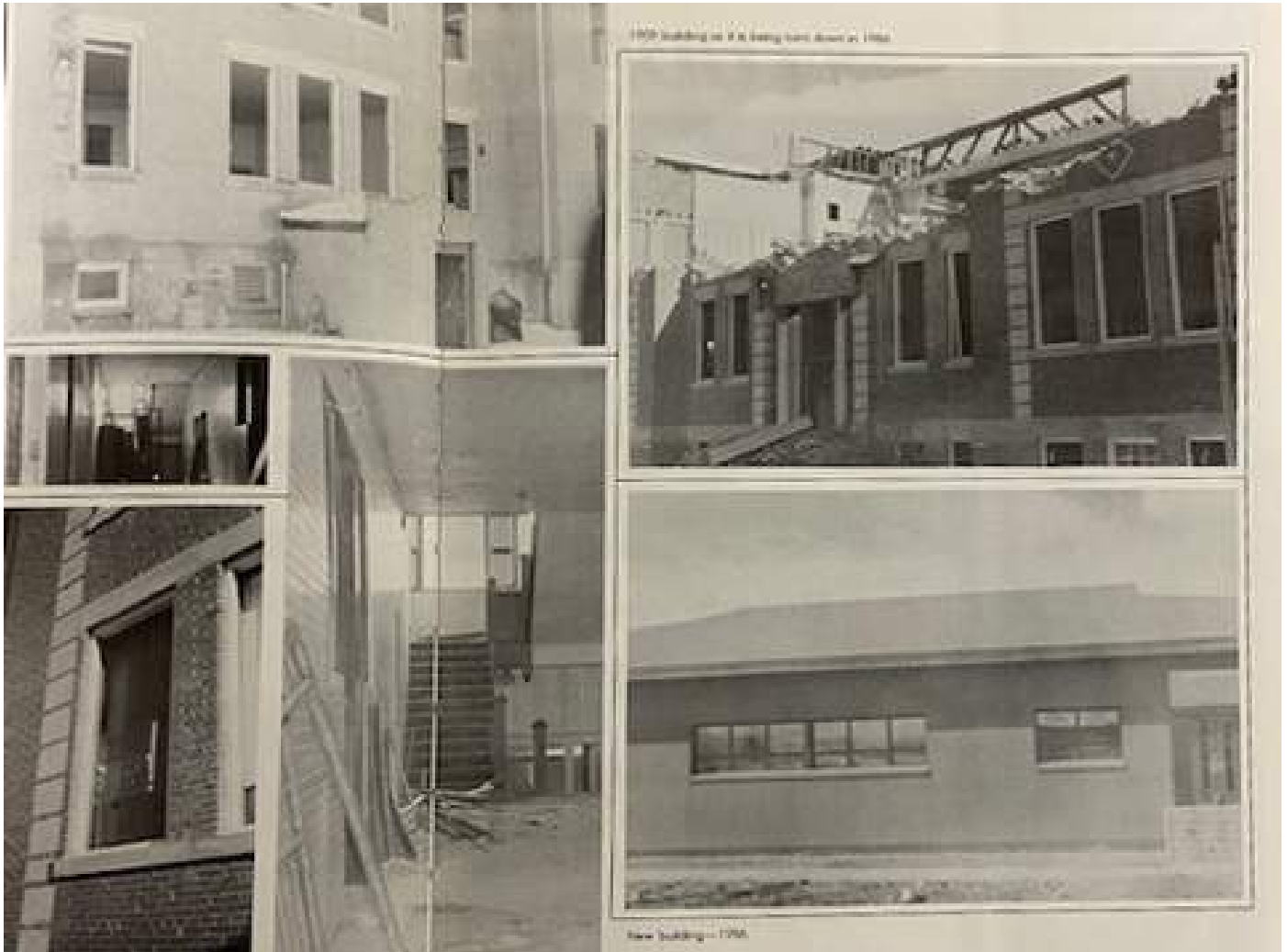
Demolition of original schoolhouse, circa 1985. (Courtesy of Jefferson High School)
