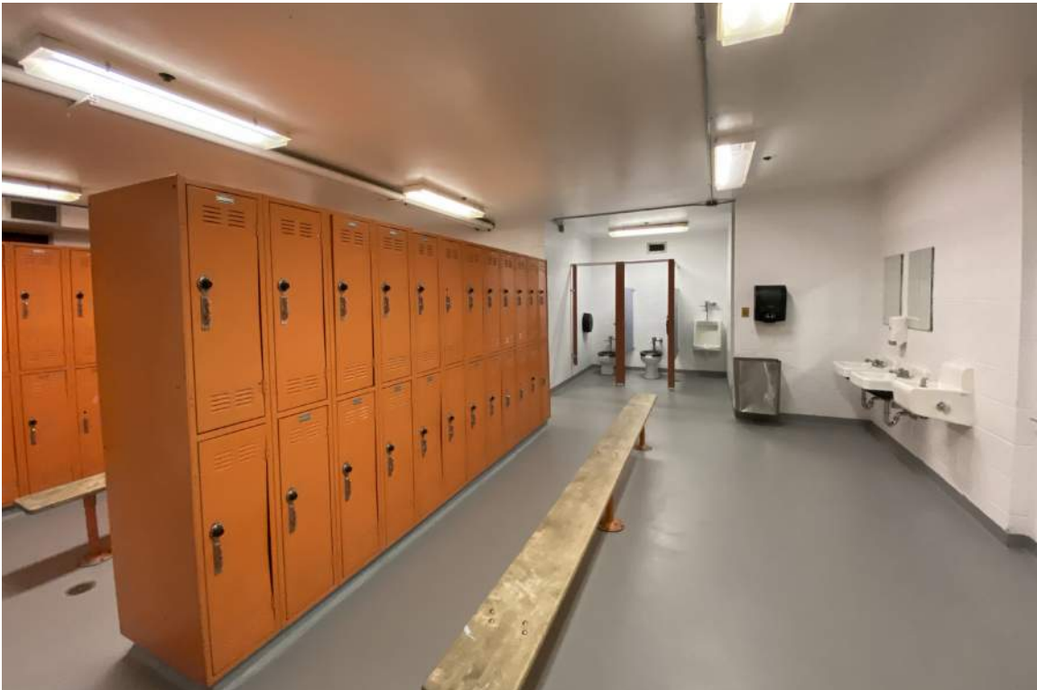
Men's locker room in the lower level of the gym. There are multiple issues in this space, such as accessibility, ventilation problems and doors missing from the stalls. Equipment storage outside this room poses potential Title IX problems.
