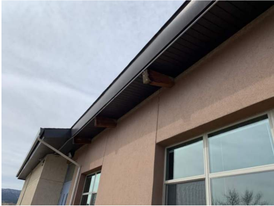
Figure 11. Exterior Ends of Trusses and Joists at Library (1985 Addition)
