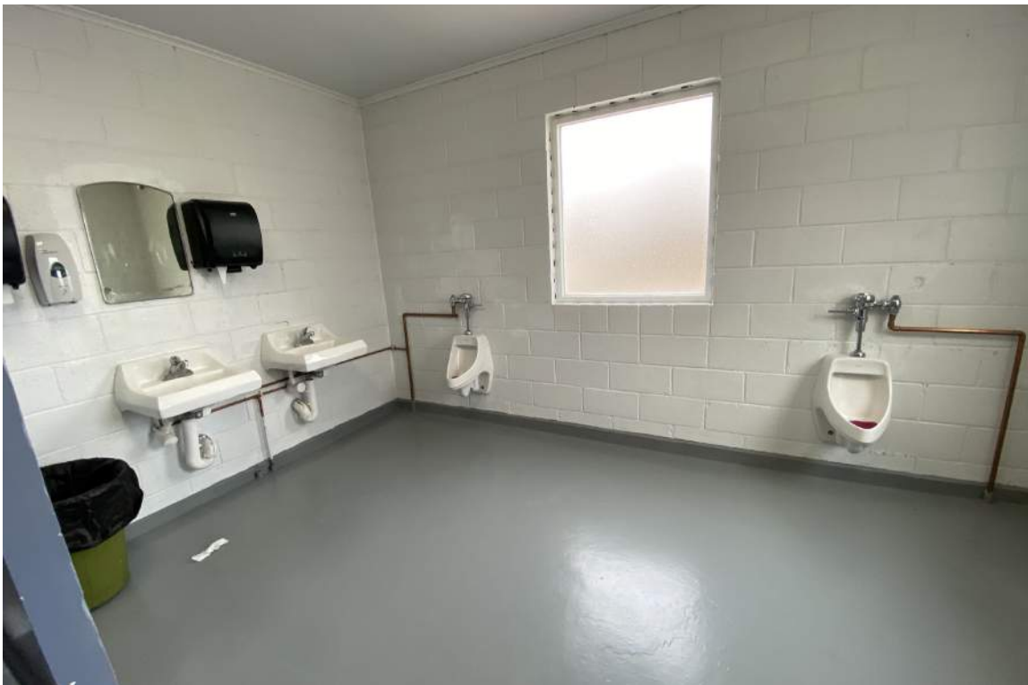
Men's restroom at the west entrance by the Existing Gym. While this room has plenty of turning and clearance space, these restrooms could be better configured to serve more students.
